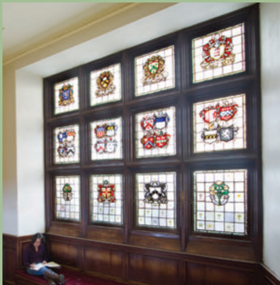
[above] Stained glass to be restored
